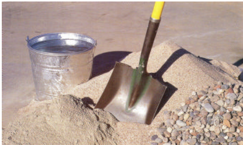
Gambar 13. Adonan beton cor
